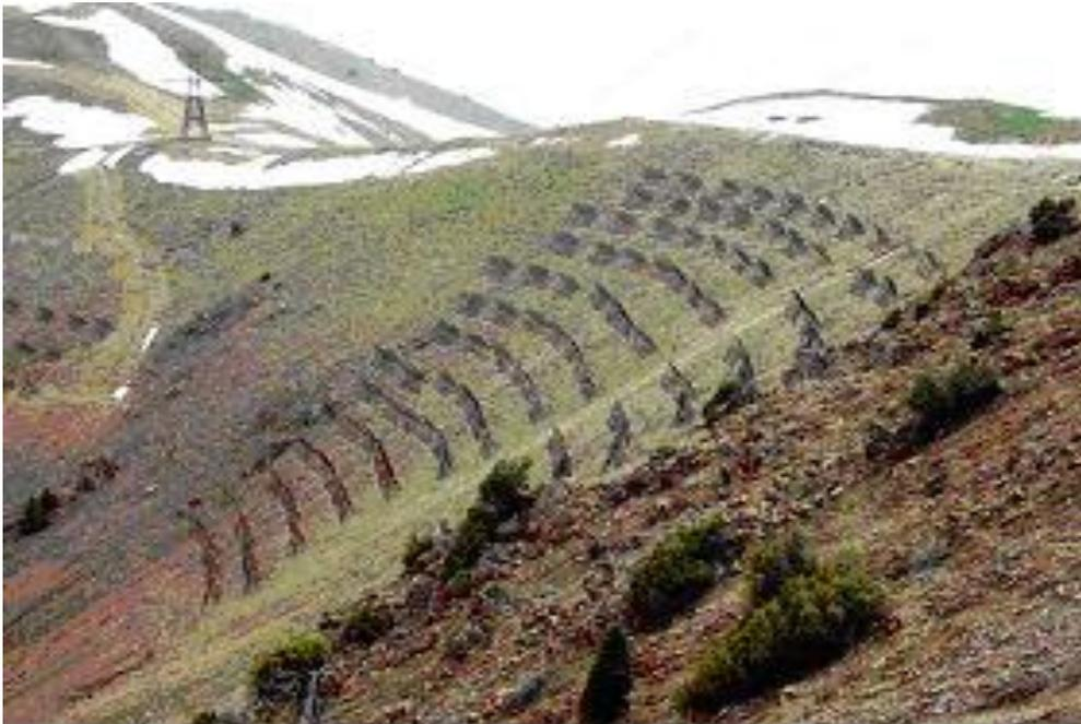
**Fig . 1.** Avalanche protection devices in the "Kamchik" pass
