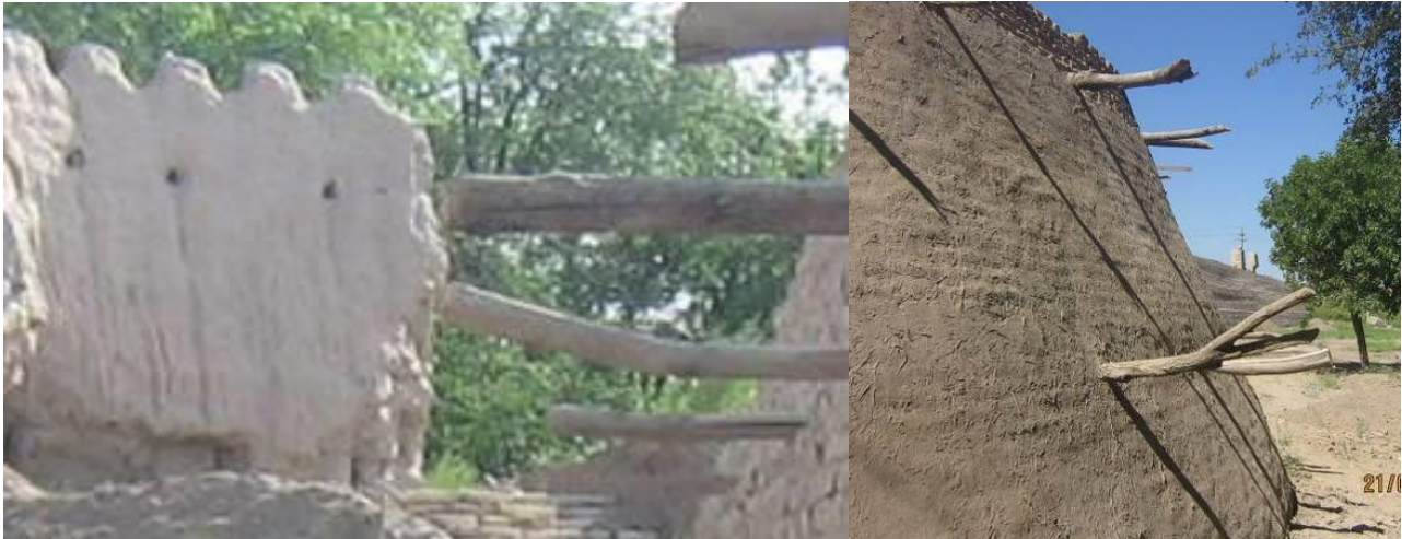
Figure 3. The usage of the wood logs in the heritage of Deshan Kala wall. (Taken by Salayev Ergash in 2013)
