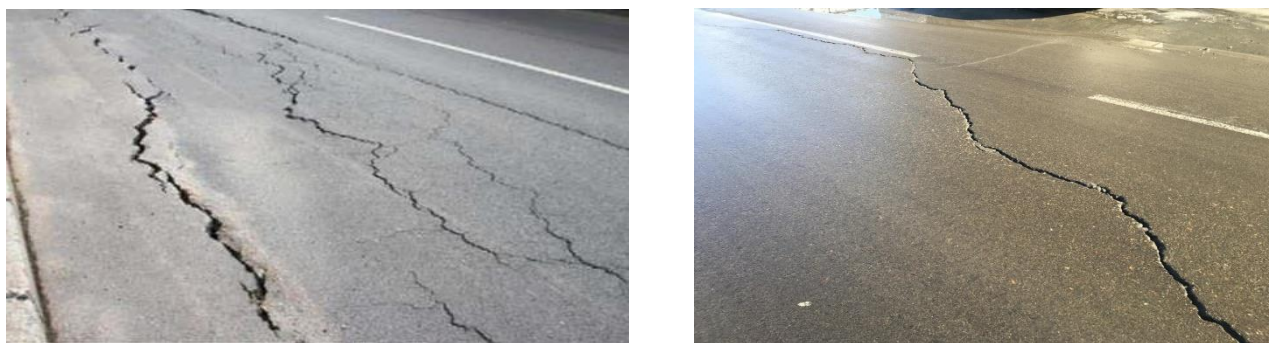
Fig. 2. Disruptions (depth) and cracks caused by deformations in the base layers of the road surface.
