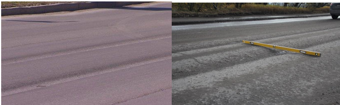
Fig. 1. Deformations of wheel tracks formed on pavements as a result of vehicle movement.
